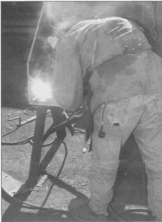
4.15 The arc spatter and radiation are dangerous. Do not allow any bystanders to observe the arc while you are welding. Also, notice how much smoke is around the welder's helmet here. The fumes are dangerous and you should have an electric fan of some kind to blow it away from you when you are welding in a corner like this.
