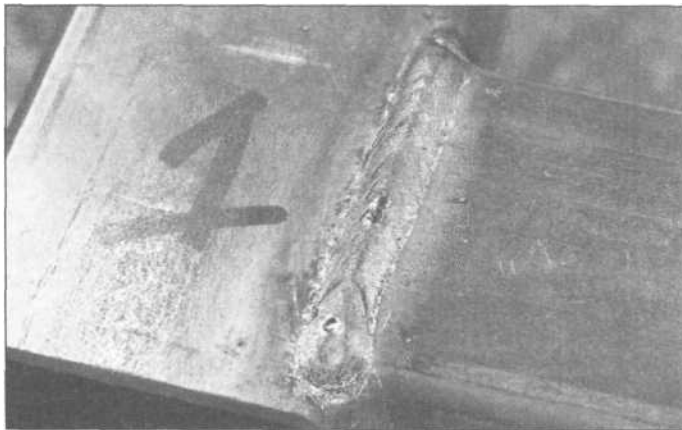
Small heat-affected zone on MIG weld
